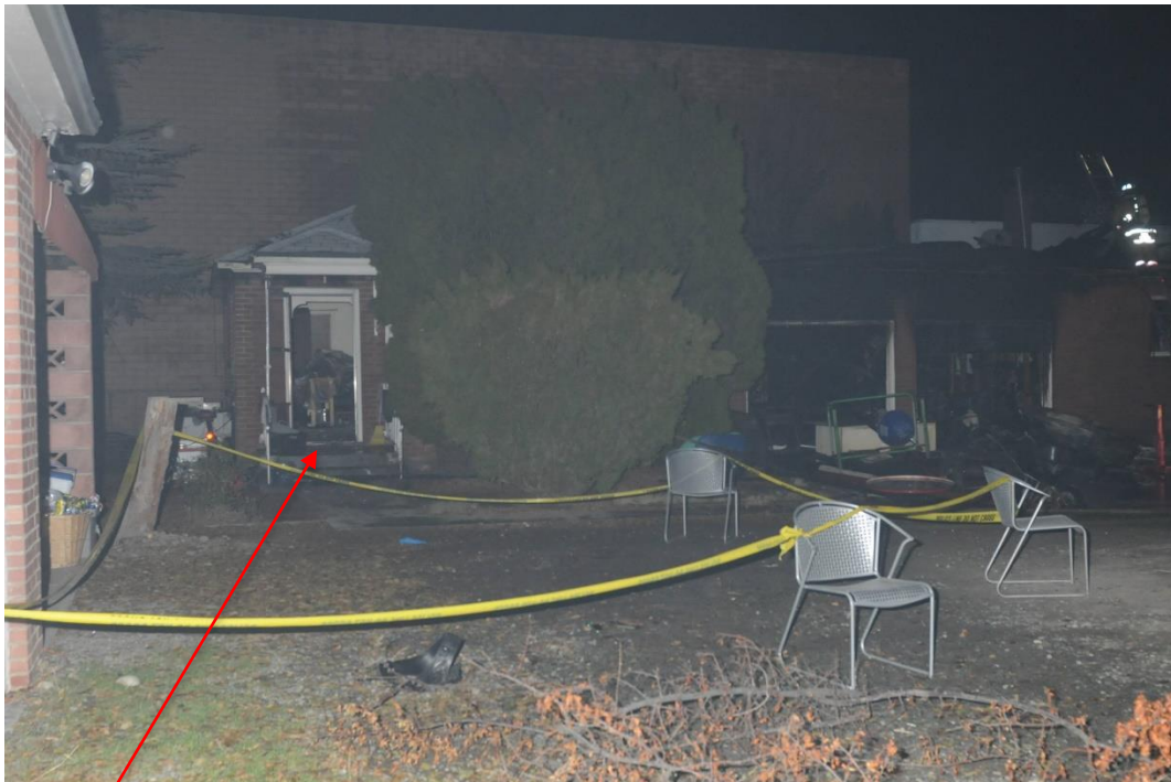
(Unit #3 at south end of driveway & garages (right side of photo) where fire believed to have originated)
